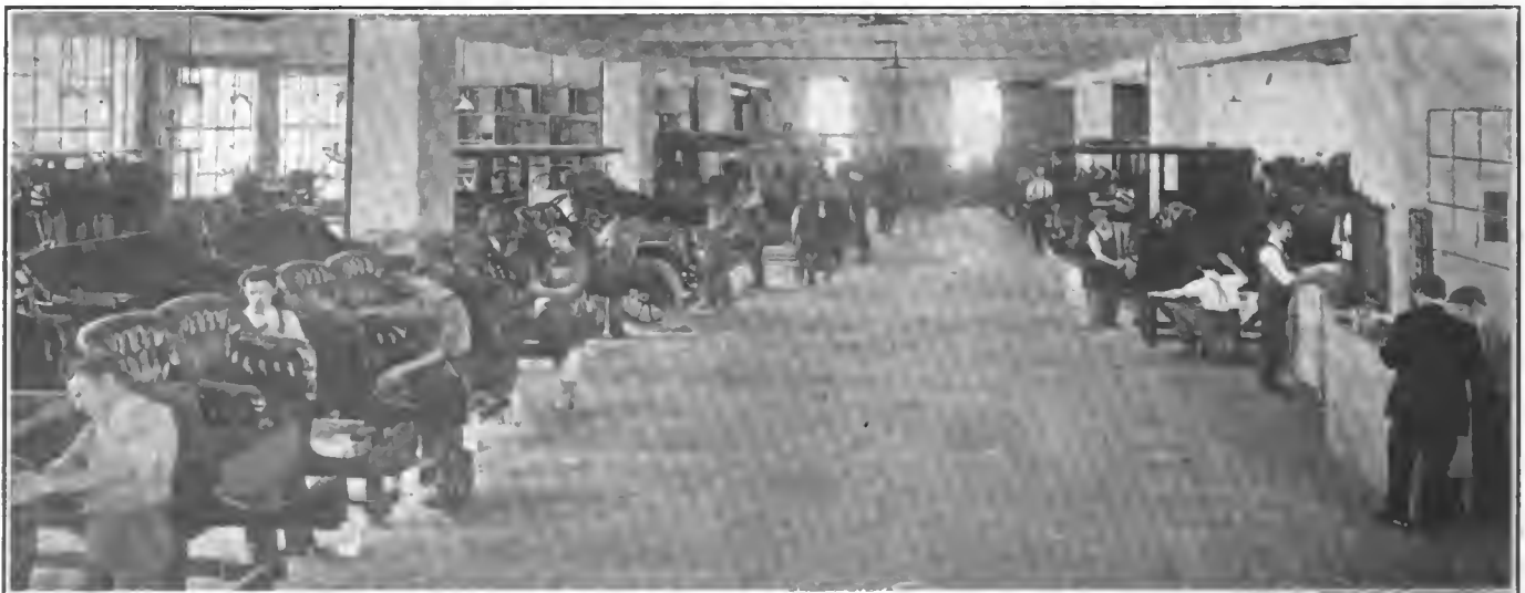
Fig. 3—A portion of the body painting department on the fifth floor. Job costs for this department are made up at the right
